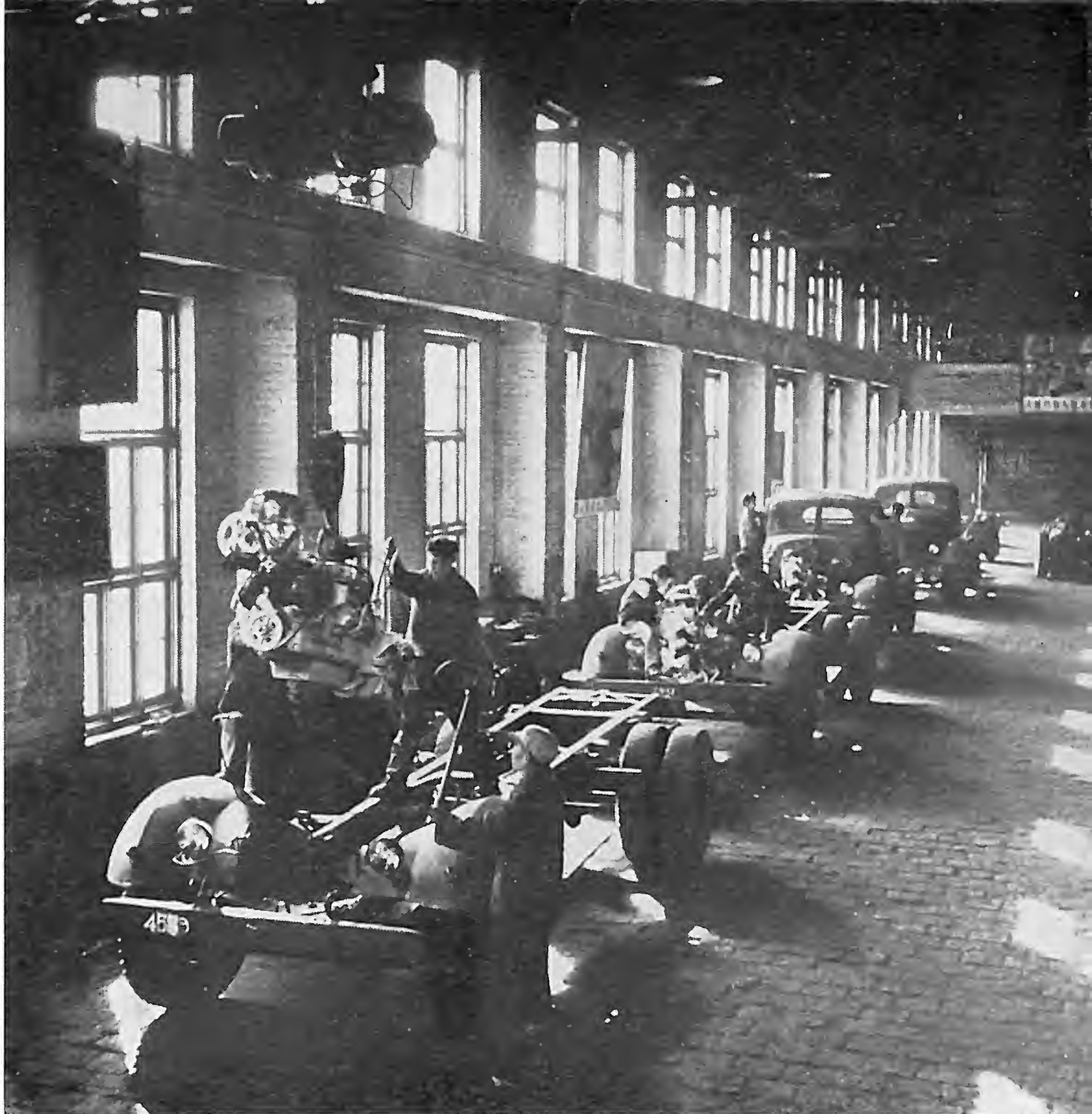
A shop in the truck repair plant.
